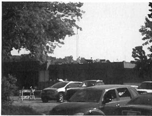
HR Annex Roof
