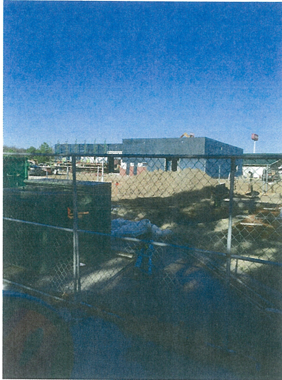
Out Post #1 Construction
