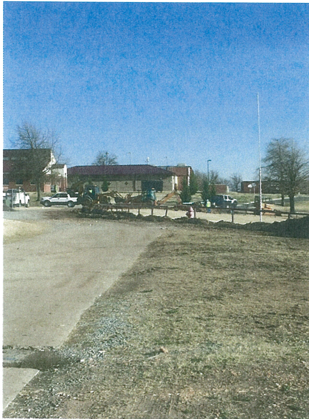
• SHS Waterline Project
