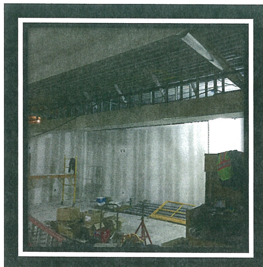
Ongoing interior upper level work
