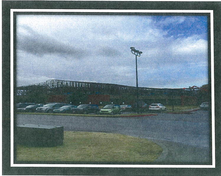
Ongoing updating roof over whole Complex
