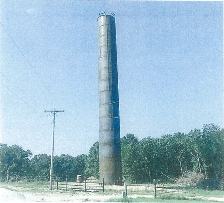
Southern Delaware Co Regional Water Project
