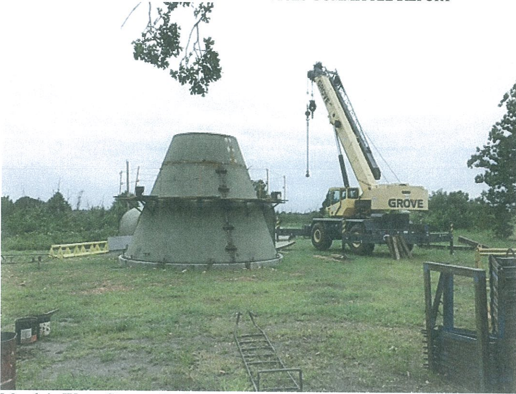
Moody's Water Storage Tank
