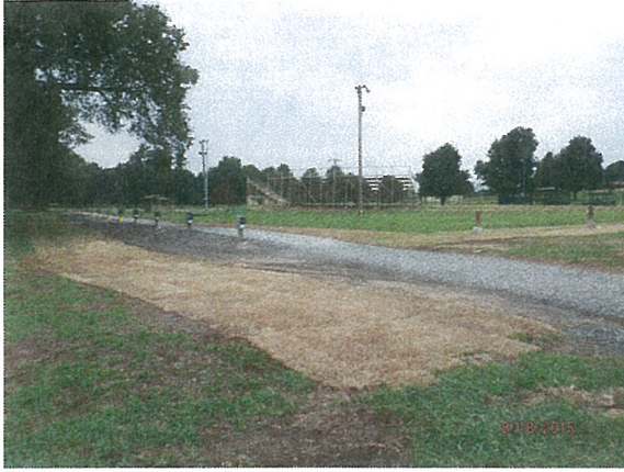
Cultural Grounds electrical improvements
