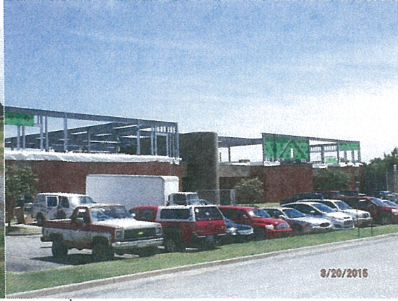
2 nd level construction on Keeler Complex
