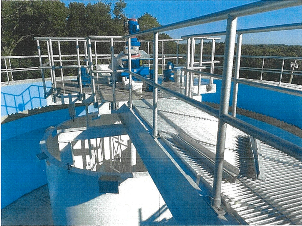
New Clarifier Locust Grove Water Treatment Plant Improvements
