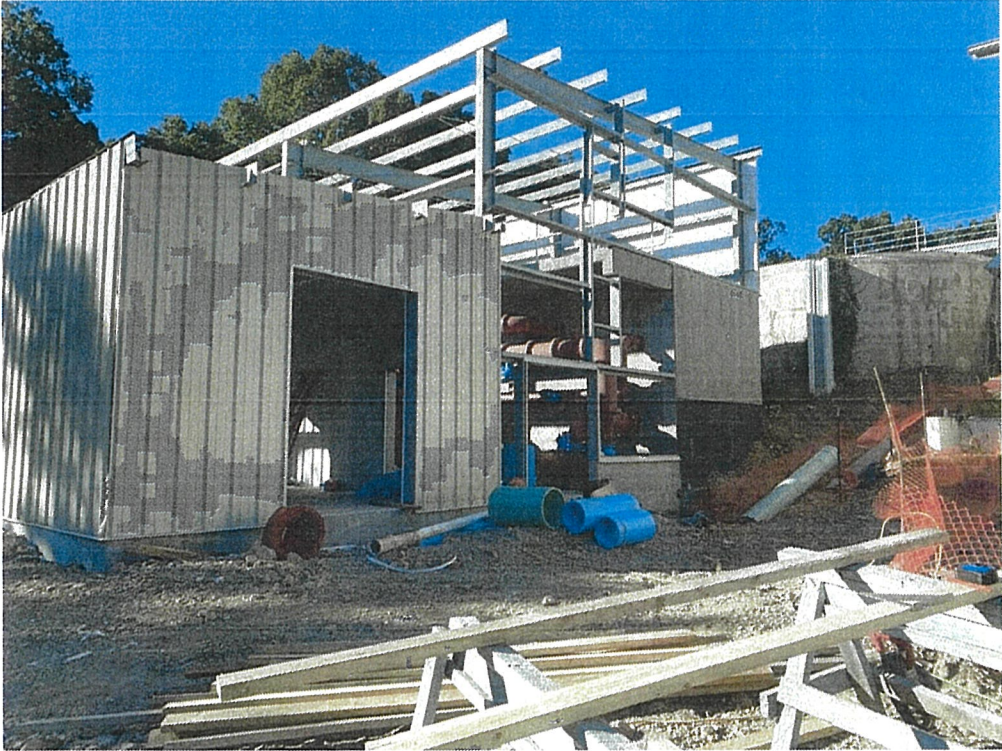
New Filtration Building Locust Grove Water Treatment Plant Improvements
