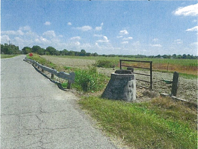
Inola WW Improvements Project
