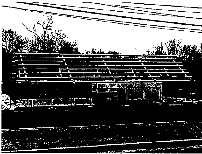
Ongoing construction - Down town Pavilion March 13, 2018
