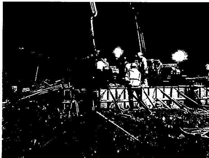
3:00 am Concrete pour – CN Outpatient Health Center March 23, 2017
