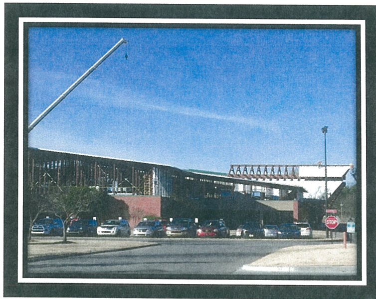
Ongoing work on upper level of Complex
