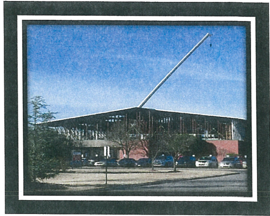
Ongoing roofing east end of Complex
