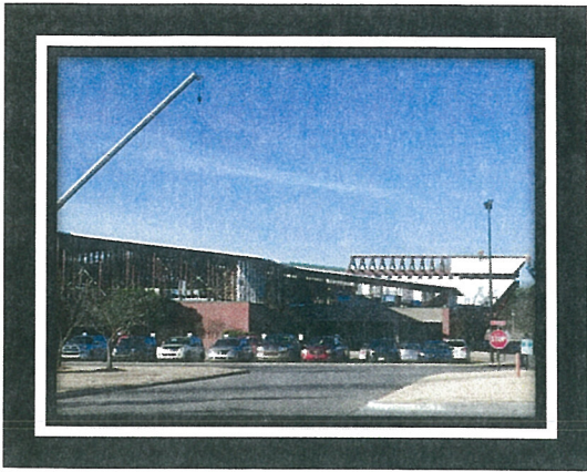
Complex installing new roof
