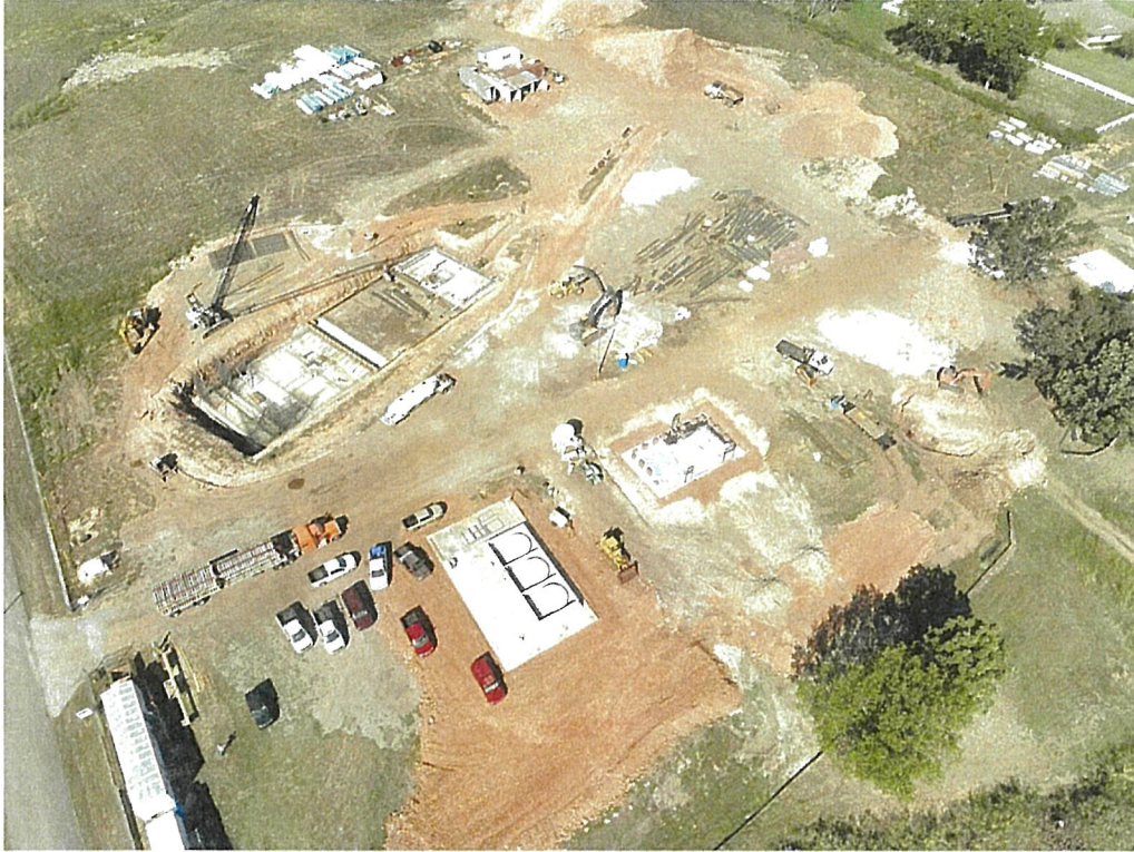
Stilwell ADA – WTP Expansion
