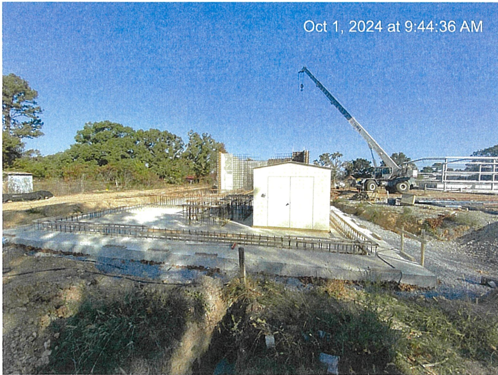
Jay PWA – WTP Expansion
