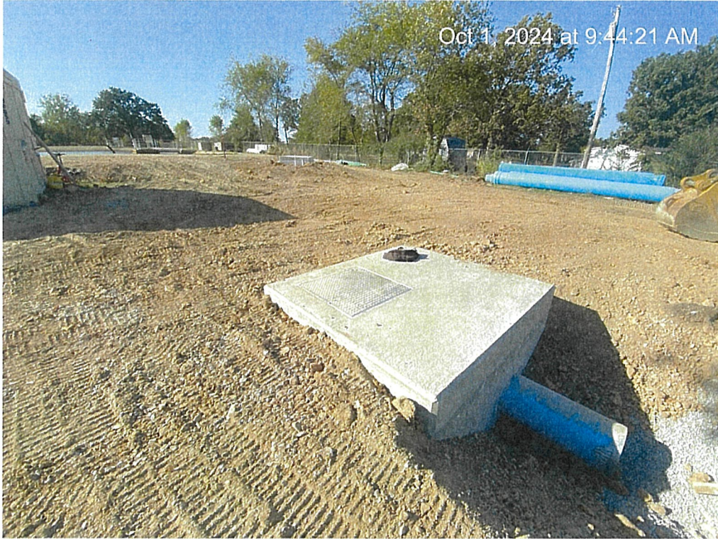
Jay PWA – WTP Expansion
