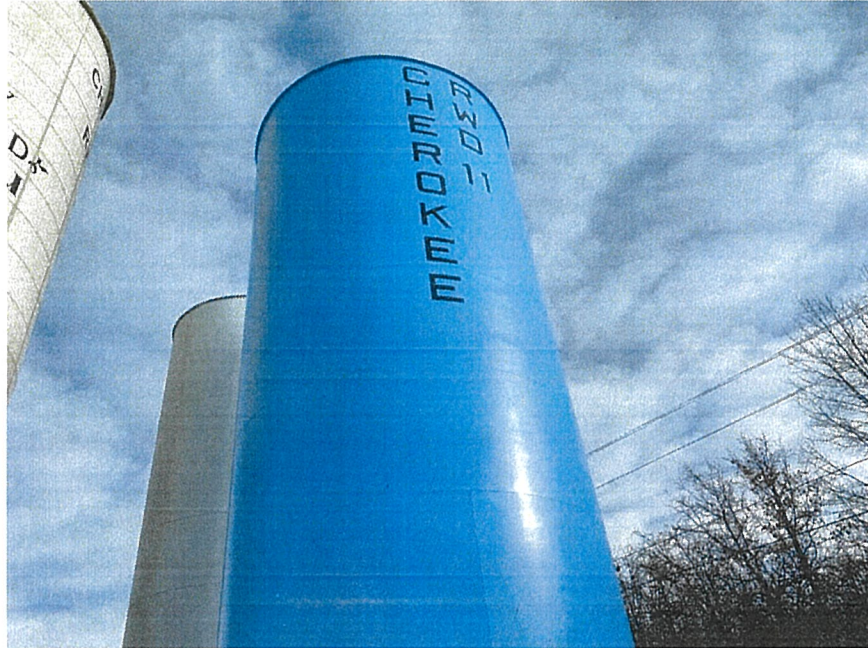
Cherokee Co RWD 11 New Tower Site
