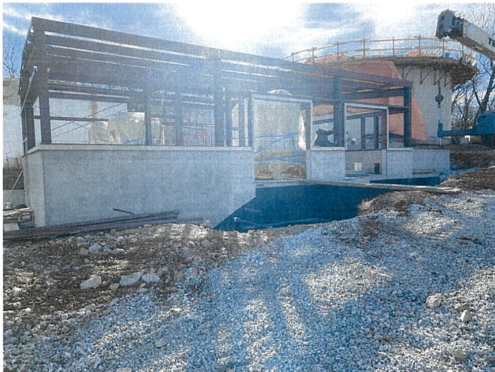
New Process Building Locust Grove Water Treatment Plant Improvements
