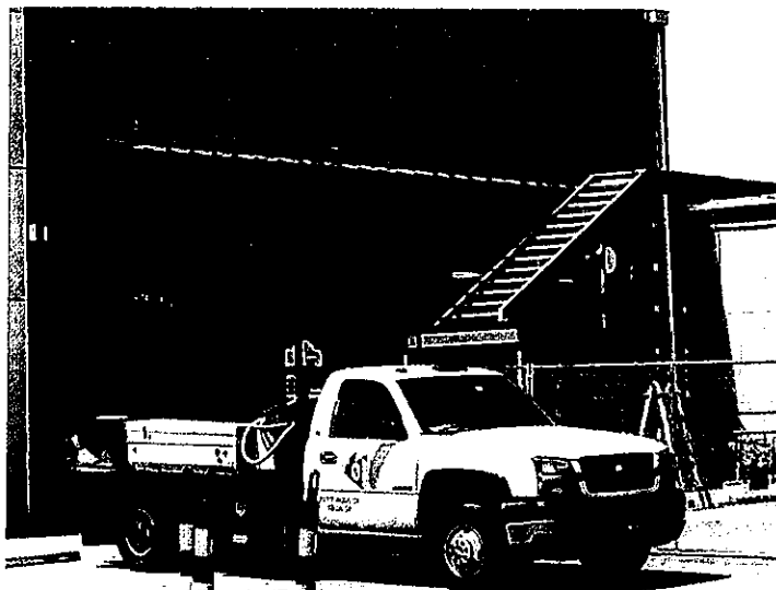
Catwalk & Stairs installed – Cort Mall April 2018
