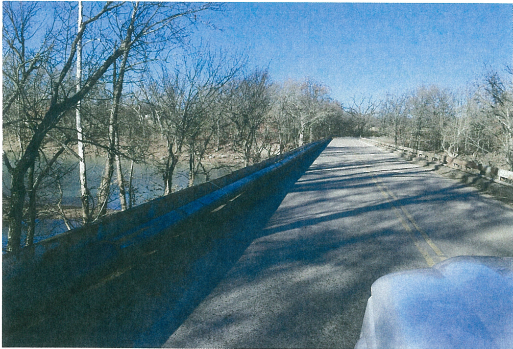
New Water Line across Barren Fork Creek – Cherokee RWD 7 Welling, OK
