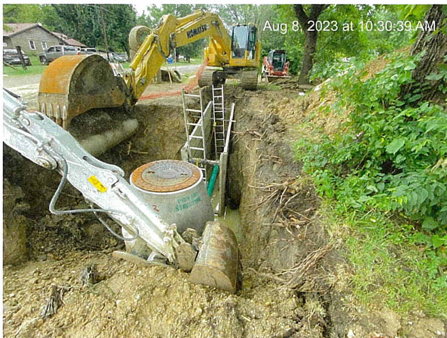
Wastewater Collection Rehab – Marble City, OK
