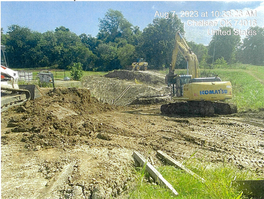
Chelsea EDA – Wastewater Treatment Plant Improvements
