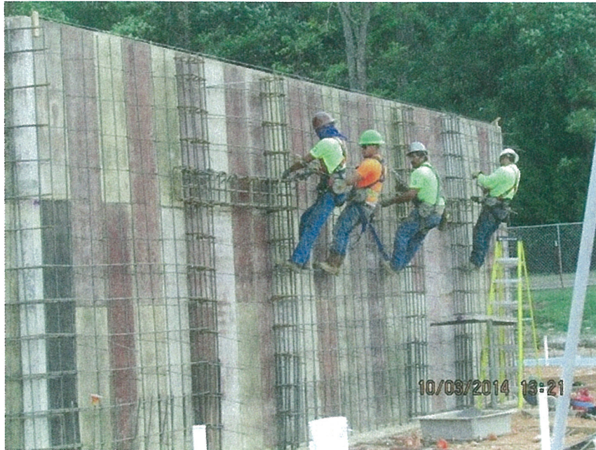
WP Mankiller Clinic Construction October 2014
