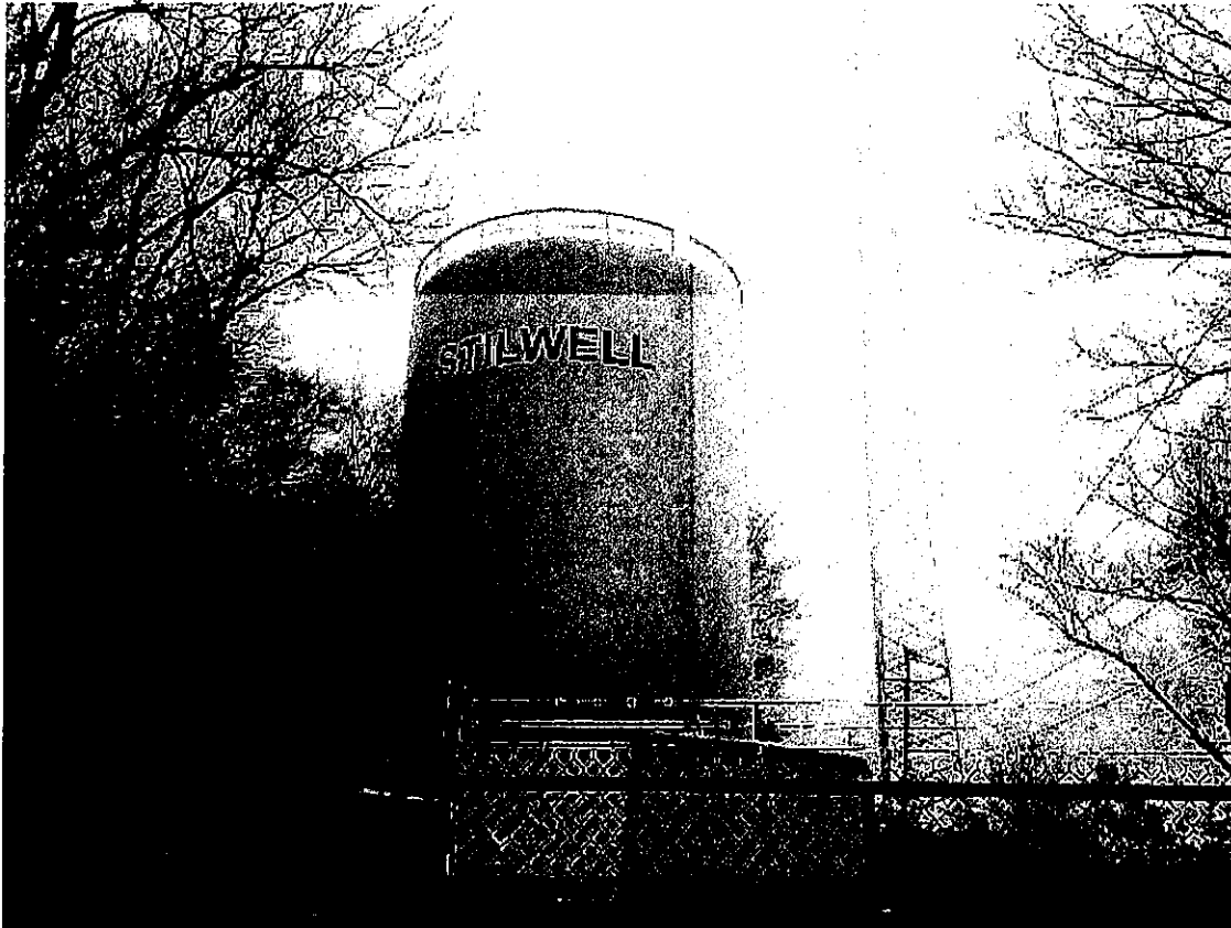
Stilwell Area Development Authority water storage tank behind the W.P. Mankiller Clinic
