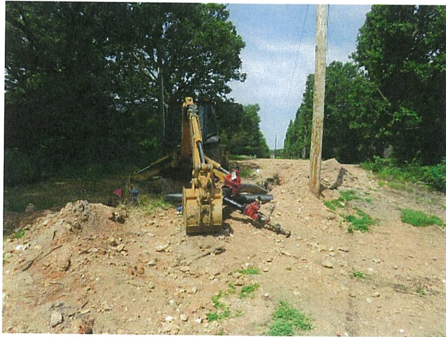
Cherokee Co RWD # 11 Improvements project.
