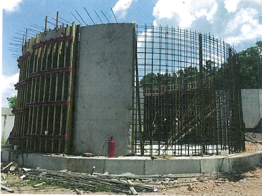
Construction of new clarifier at Locust Grove WTP.
