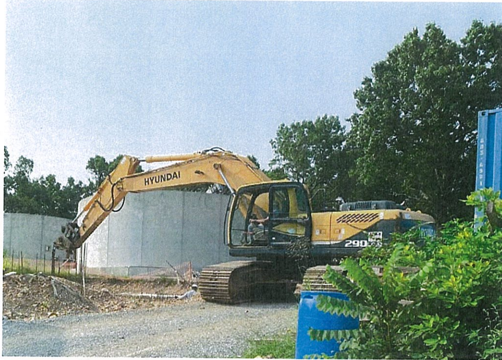
Construction of new clarifier at Locust Grove WTP.
